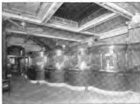
Bank Counter from the Main Entrance.
